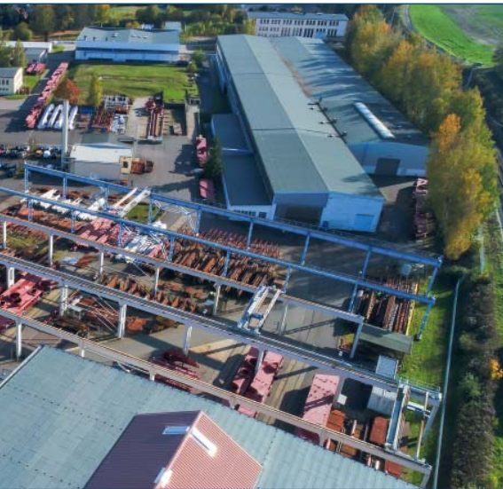
View of Meeraner Dampfkesselbau's site.
